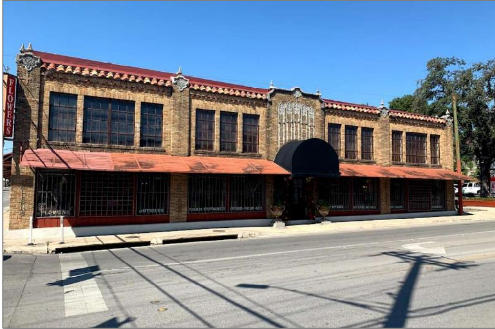
The Allen | San Antonio, TX Envelope • LED Lighting • HVAC Assessment: $1,559,719 Capital Provider: PACE Equity, LLC
