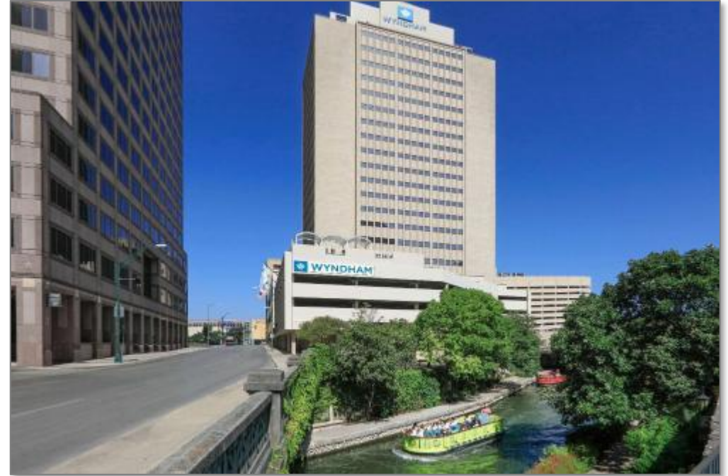
Intercontinental Hotel | San Antonio, TX Envelope • Plumbing • LED Lighting • Water Conservation • HVAC Assessment: $28 million Capital Provider: Nuveen Green Capital
